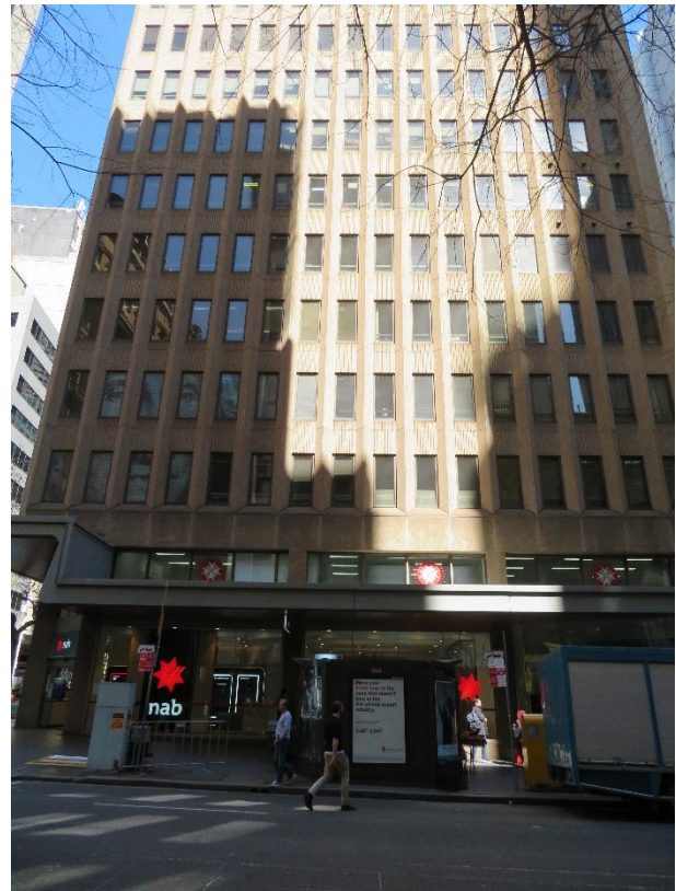
Figure 26 Currency House (northern Hunter Street façade)
