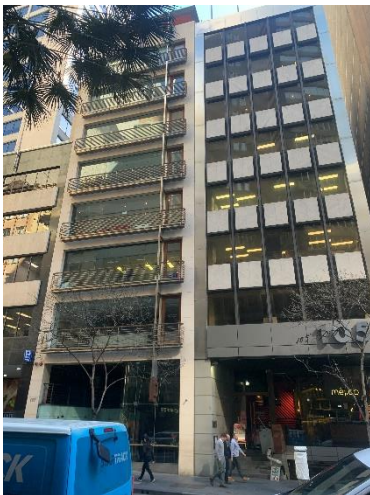
Figure 31 The principal façade, showing the contemporary refurbished façade
